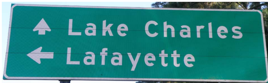
Figure 2D.7.2 Example of DOTD Destination Sign with Arrows
